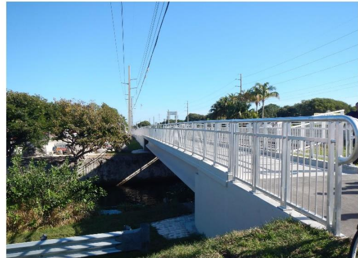
Monroe County – Marvin Adams Pedestrian Bridge
